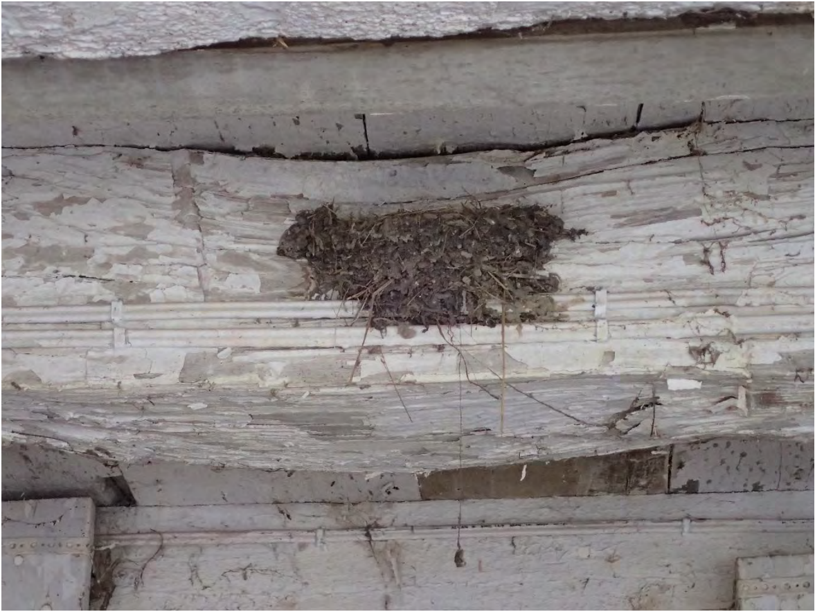
Photo 3. Barn swallow nest on beam in lower level of barn.
