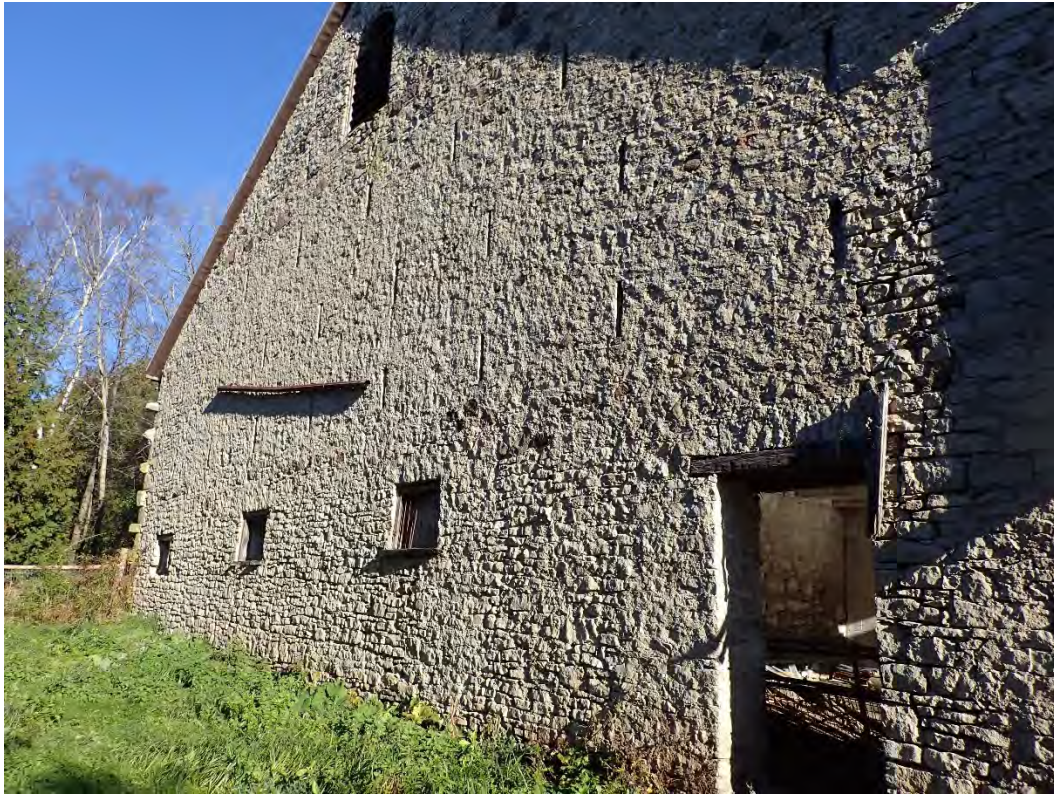
Photo 4. Exterior stone wall of barn.
