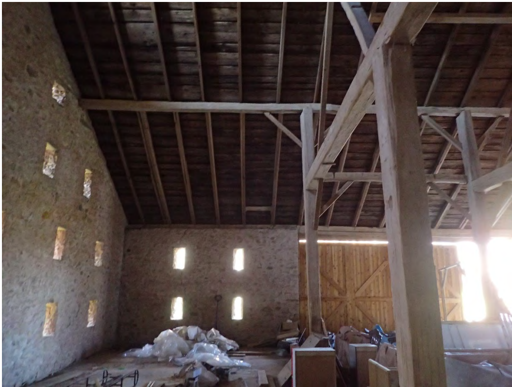
Photo 5. Interior, main level of the barn.
