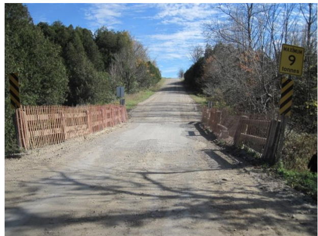
Photograph 12 ↑ Bridge structure – view of bridge from 3 rd Line West
