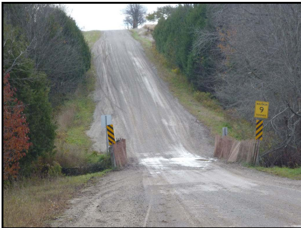
Plate 7: View of Lands Sloped > 20°, Southeast of Bridge (Facing Southeast)
