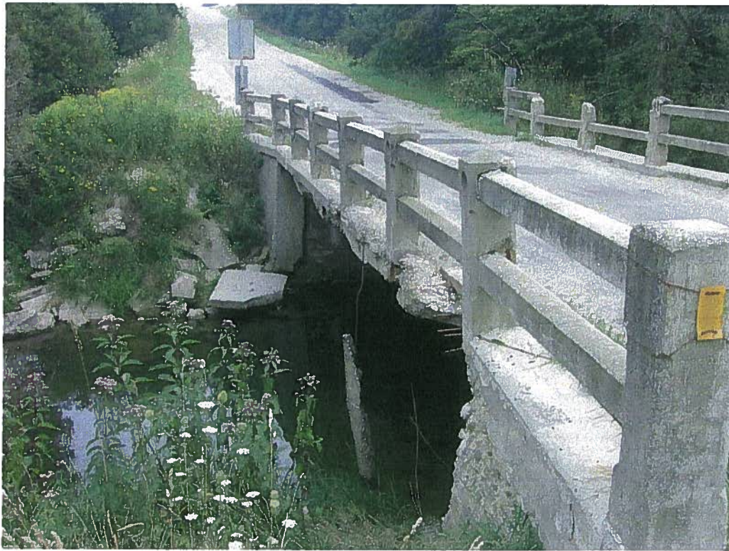
Photo 2: Looking at east side of bridge.
