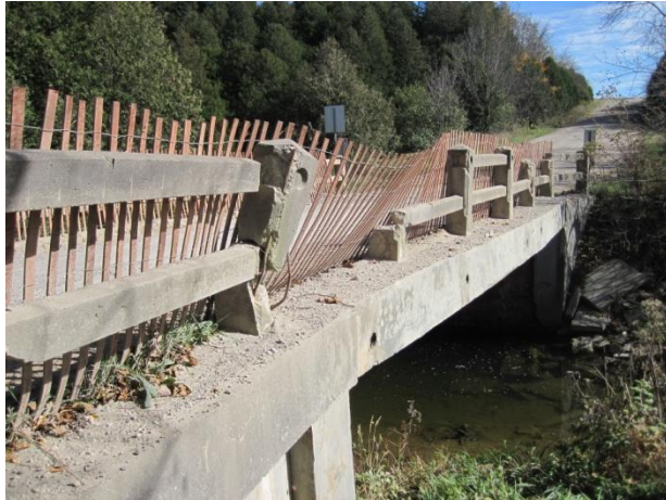
Photograph 13 ↑ Bridge structure – downstream side
