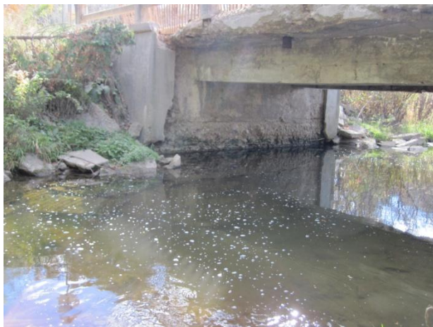
Photograph 11 ↑ Bridge structure – upstream side view of pool under bridge
