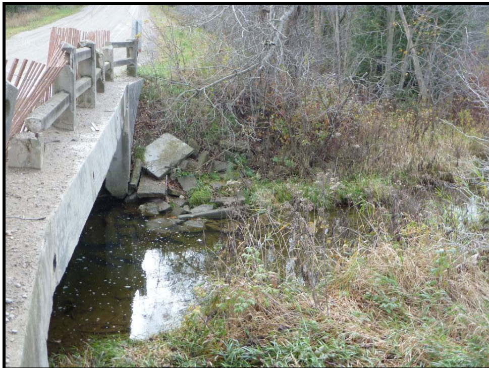
Plate 6: View of Lands Sloped > 20° on West Side of Bridge (Facing Southeast)
