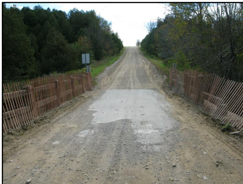
Plate 1: 3 Line West at Carroll Creek Bridge looking south.
