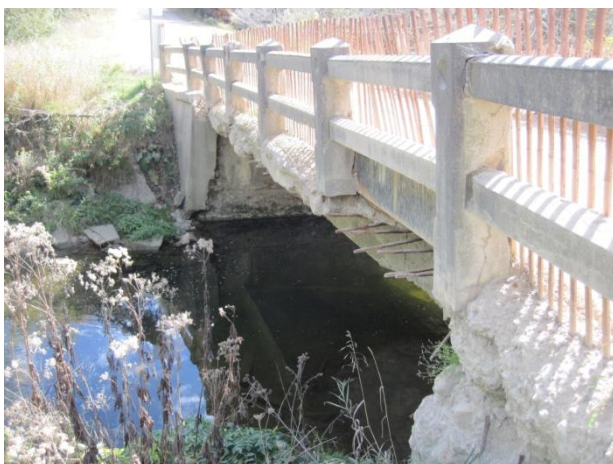
Photograph 8 ↑ Bridge structure – upstream side
