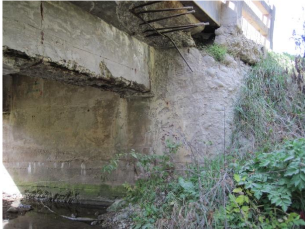
Photograph 9 ↑ Bridge structure – upstream side left bank
