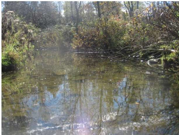
Photograph 15 ↑ Downstream Reach – facing downstream from bridge
