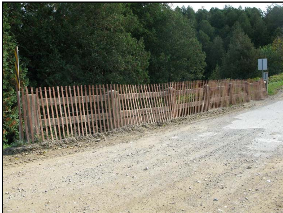
Plate 12: Snow fencing lining the east railing of Carroll Creek Bridge.
