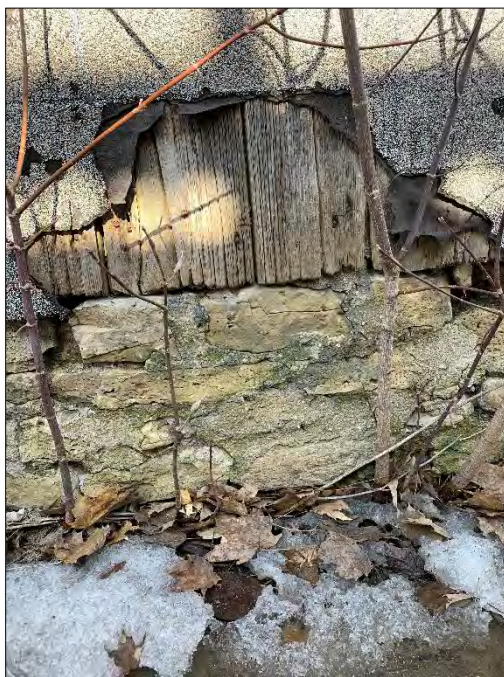
Figures 34, 35, 36 & 37: (above left) View of south elevation of outbuilding; (above right) View of south and east elevation; (below left) View of limestone foundation and wood cladding below insulbrick; (below right) View of interior of outbuilding (Source: MHBC, 2021).
