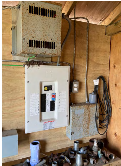
Photo 6 – View inside the maintenance shed.
