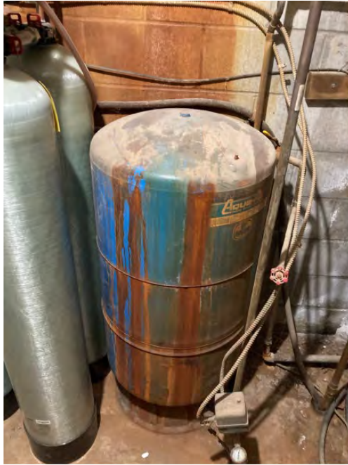
Photo 3 – View in the furnace room in the residence.
