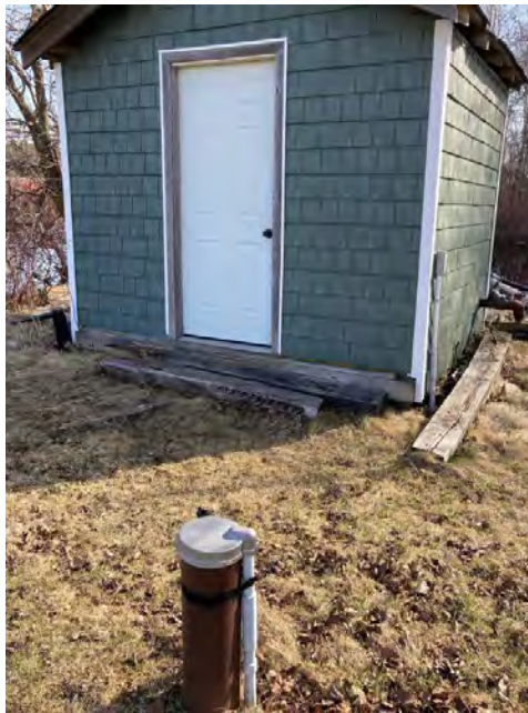
Photo 5 – View looking east towards maintenance shed with domestic water well.
