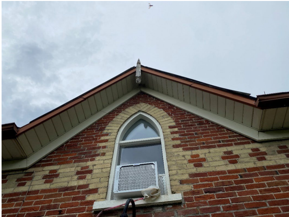
Photo 12: View of wood framed gothic arch window.
