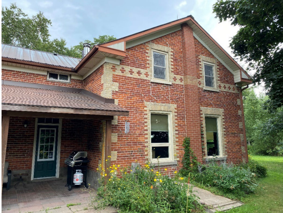
Photo 3: View of south west elevation.
