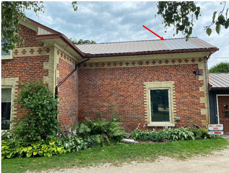
Photo 8: View of metal roofing and replaced panel section.
