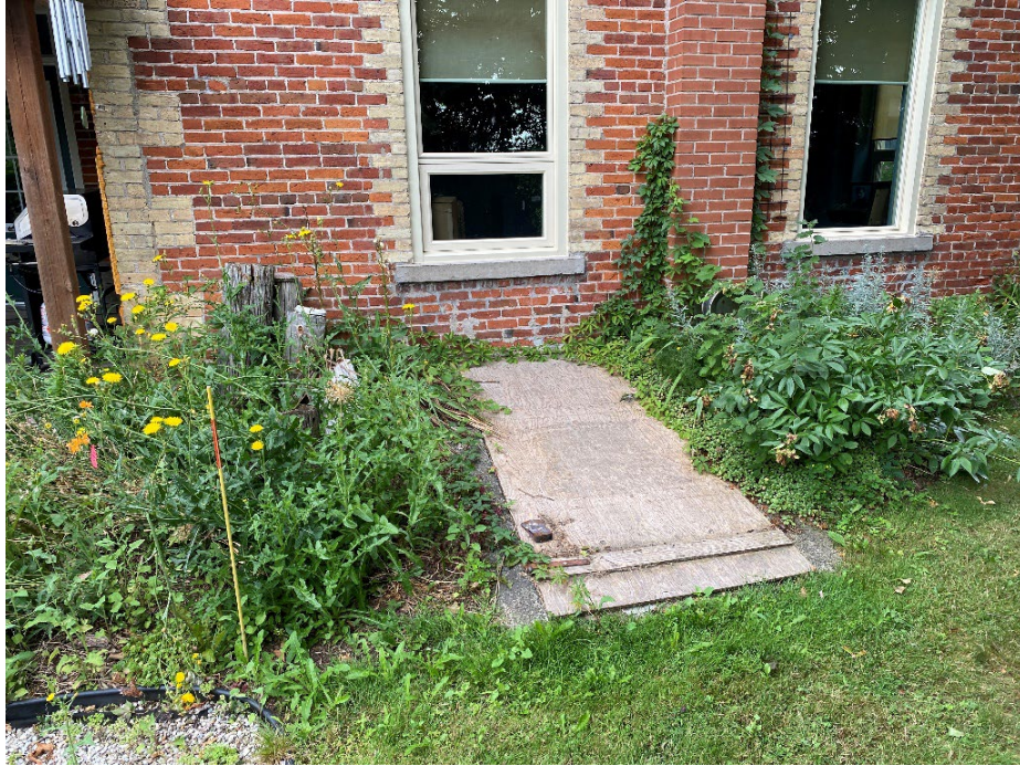
Photo 11: View of windows, basement hatch.
