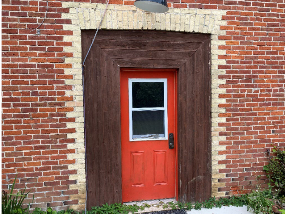
Photo 13: View of front door with infilled wood cladding.
