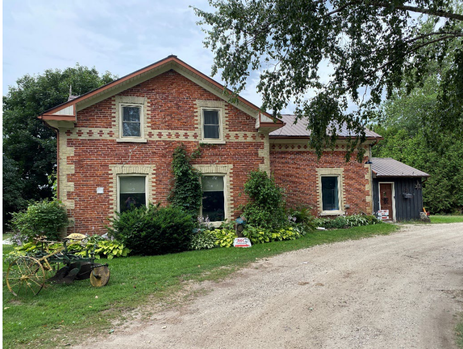
Photo 1: View of north east elevation.
