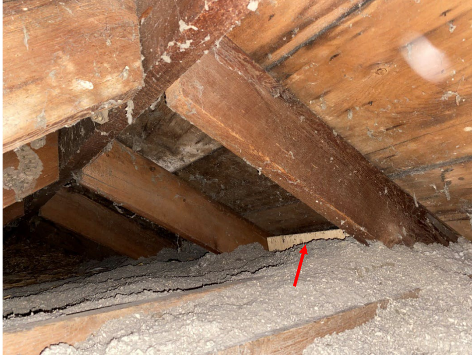
Photo 7: View of attic insulation, likely bulkhead for soffit ventilation.
