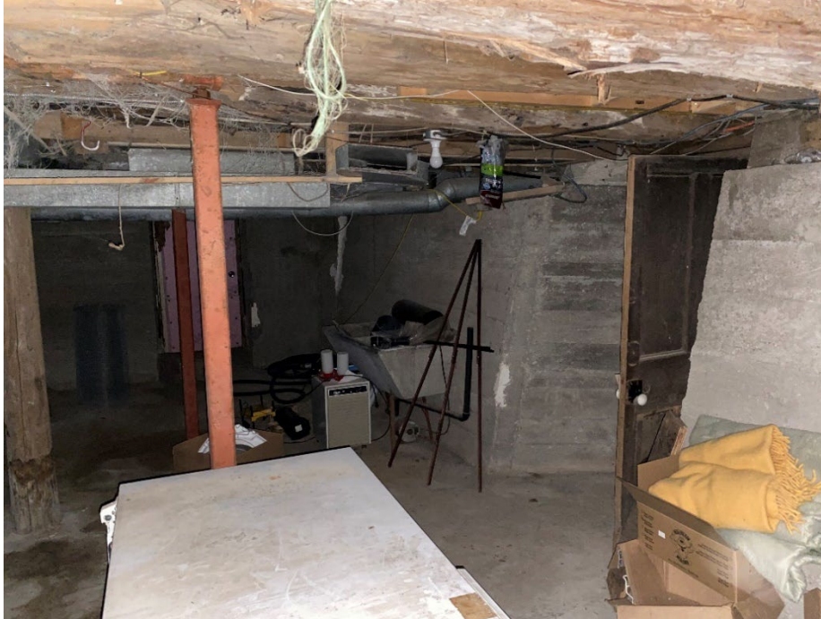
Photo 5: View of concrete foundation angle, wood and steel post supports.
