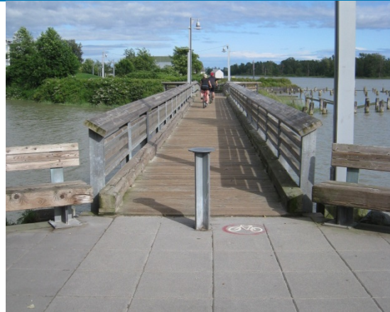
Lower Right: Centre Bollard Over Trail Bridge, Steveston, BC Source: MMM Group
