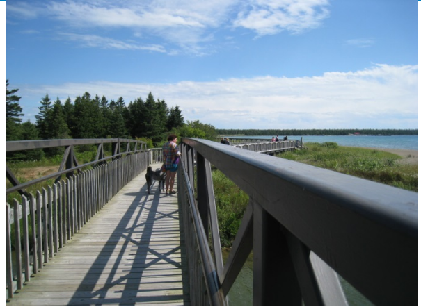
Providence Bay, ON Source: MMM Group
