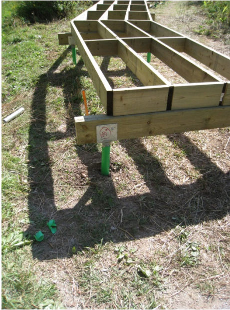
Low Profile Boardwalk on Helical Piles Foundation, Halton Hills (Georgetown) ON.
