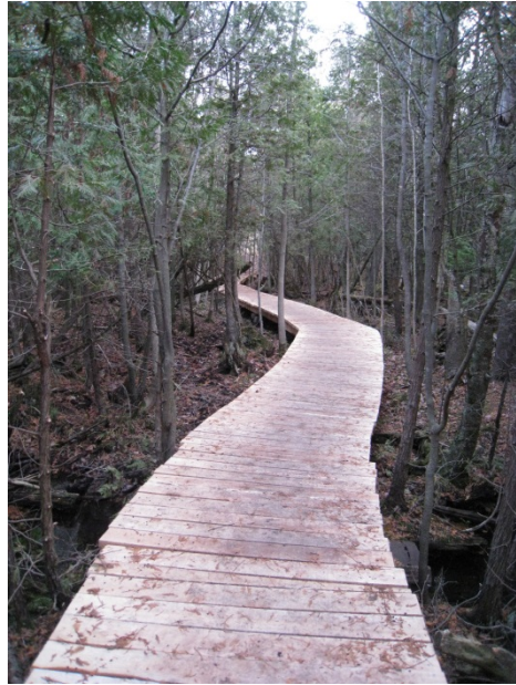
Low Profile Boardwalk on “Deck Block” Foundation, Guelph ON.
