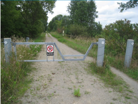
Heavy Duty Swing Gate, near Orton, ON. Source: MMM Group
