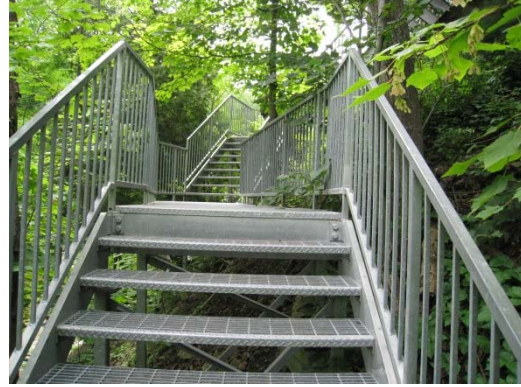
Metal Mesh Trail Stairway System, Kagawong, ON.
