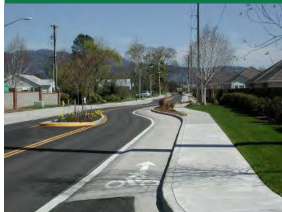
Example of a Raised Bicycle Lane on Ayres Road Source: "Cycle Tracks: Lessons Learned", Alta Planning + Design 2008
