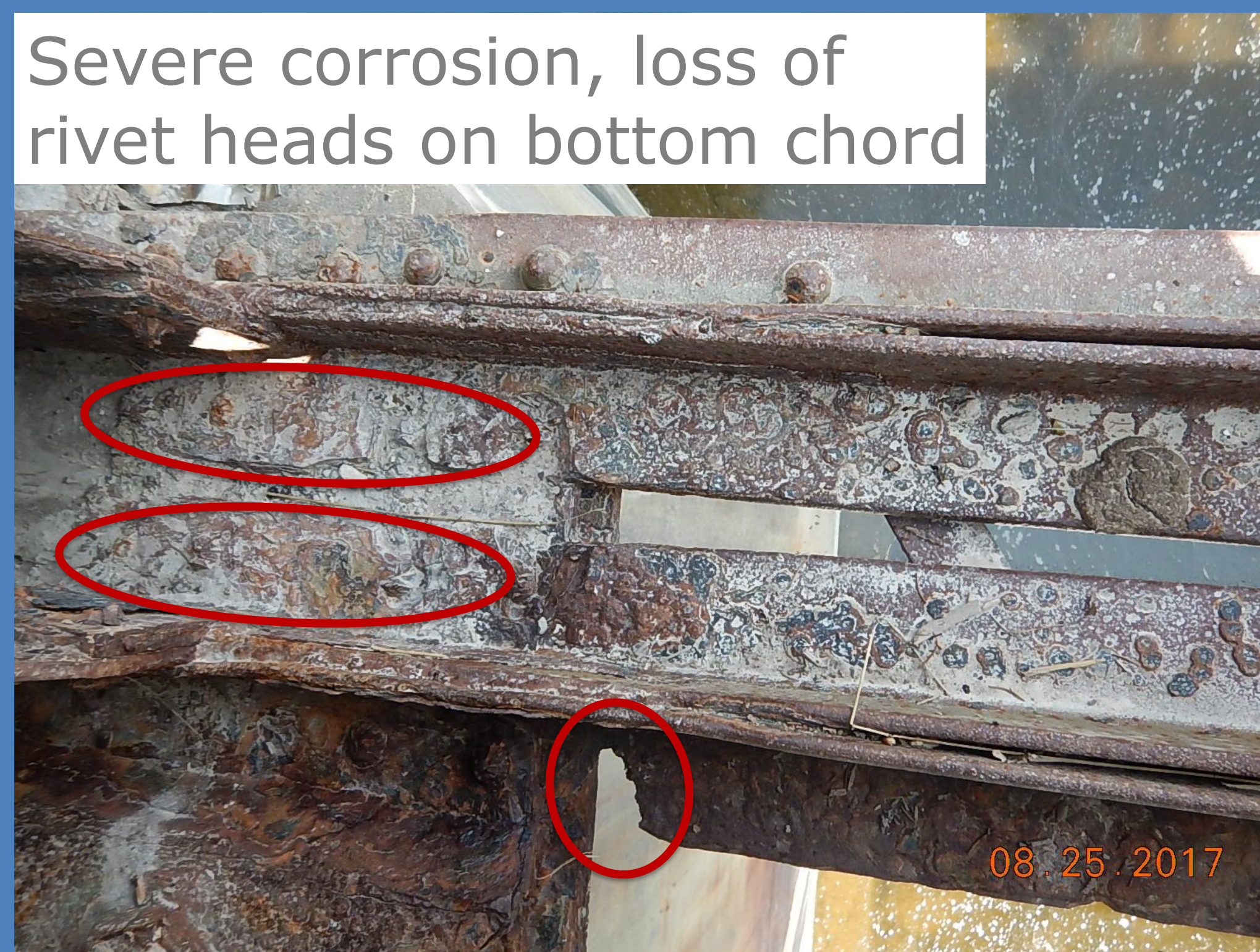
Stringers with severe corrosion and perforations
