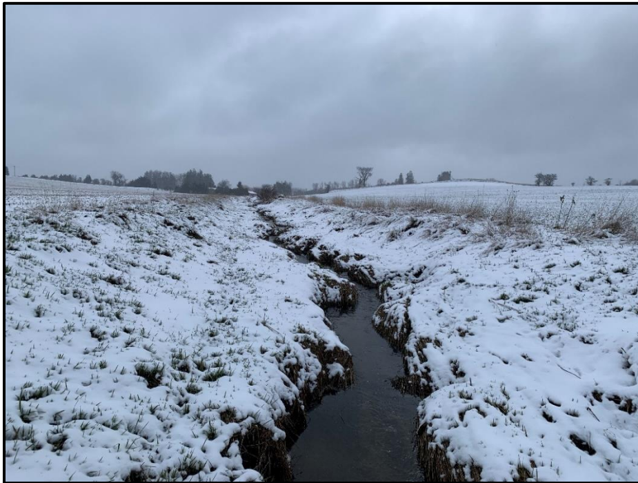
Photograph 3. A View of The Upstream Portion of the Nichol Drain. Facing Upstream (April 19, 2022)
