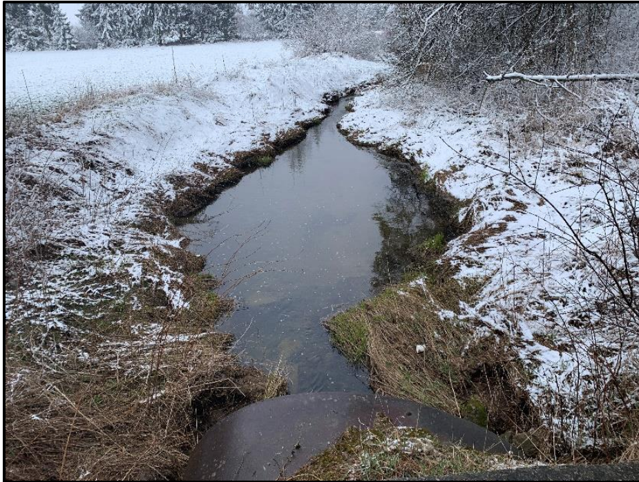
Photograph 5. The Pool Immediately Downstream of The Driveway Culvert. Facing Downstream (April 19, 2022)
