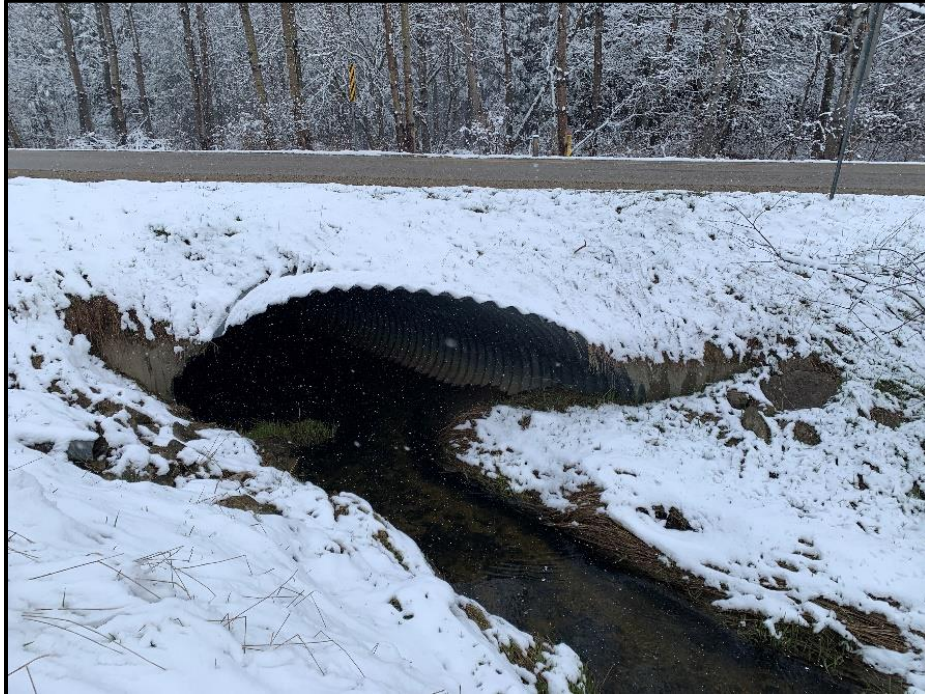
Photograph 2. Steel Pipe Culvert Traveling Under Sideroad 15. Facing Downstream (April 19, 2022)
