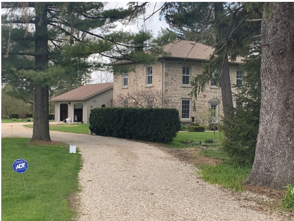
Figure 15: Current view, looking north-west towards the two storey house (Source: MHBC, 2021)
