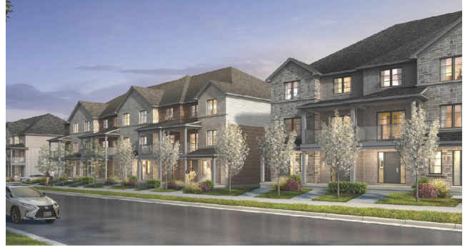
Example of facade variety in townhouse developments.
