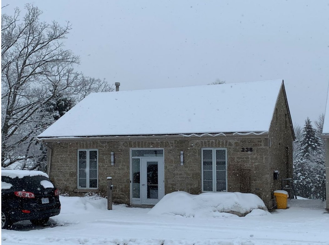
Figure 28: 238 St Patrick Street E in current condition (MHBC, 2022)
