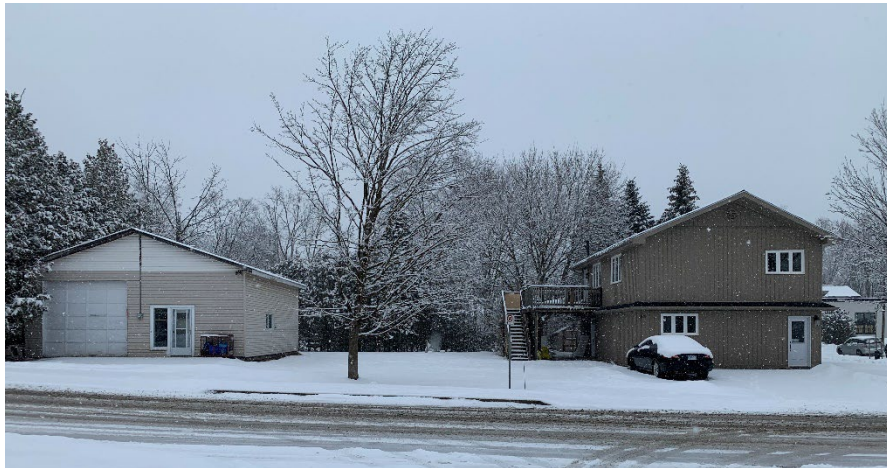
Figure 3: Street view of subject property from Gowrie St (Source: MHBC, 2022).
