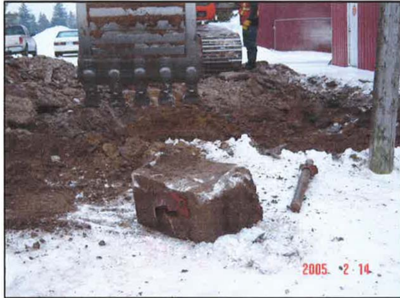
Photo 3 Concrete block and post uncovered at 1.2 mbgs
