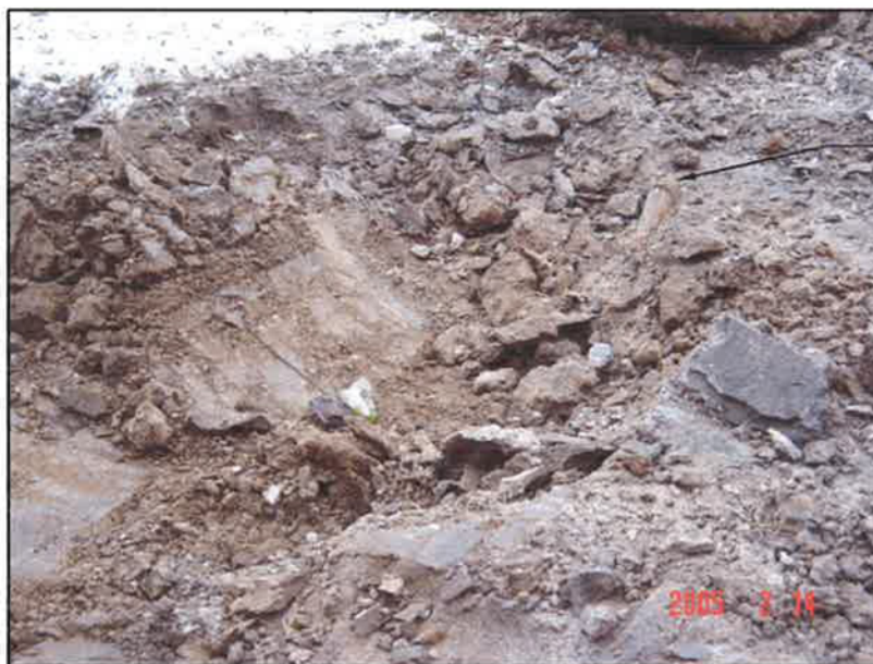
Photo 2 Fill pipe uncovered at 0.8 mbgs
