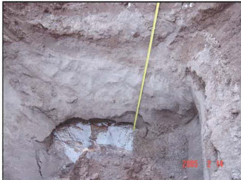
Photo 4 Northeast wall of excavation
