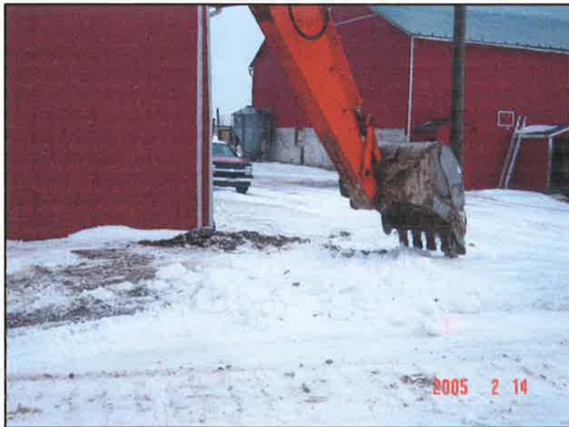
Photo 1 Location of former UST
