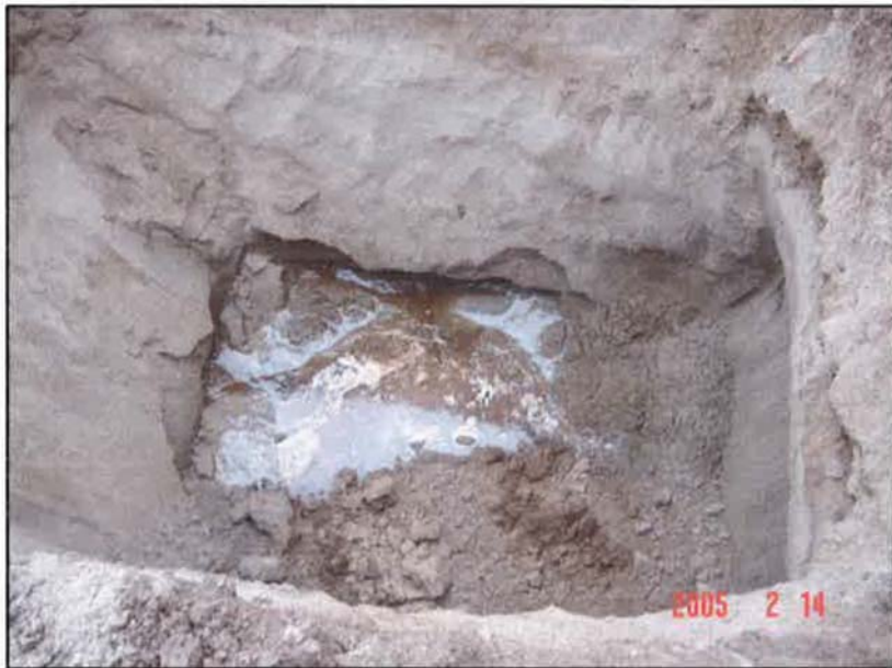
Photo 5 Bottom of excavation Water table intersected at 2.8 mbgs
