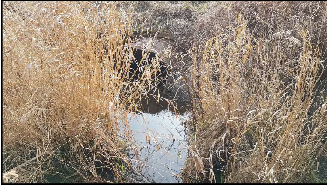
PHOTOGRAPH NO.: 25 FROM: Confluence of all three reaches LOOKING: onto culvert
