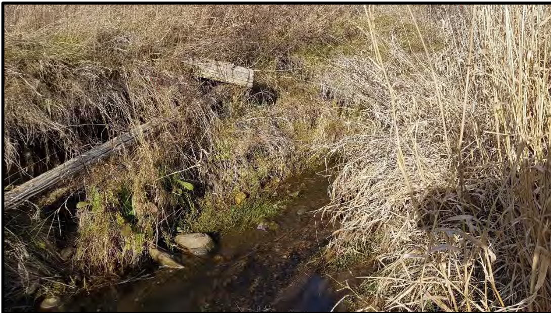
PHOTOGRAPH NO.: 16 FROM: Centre of creek LOOKING: Downstream
