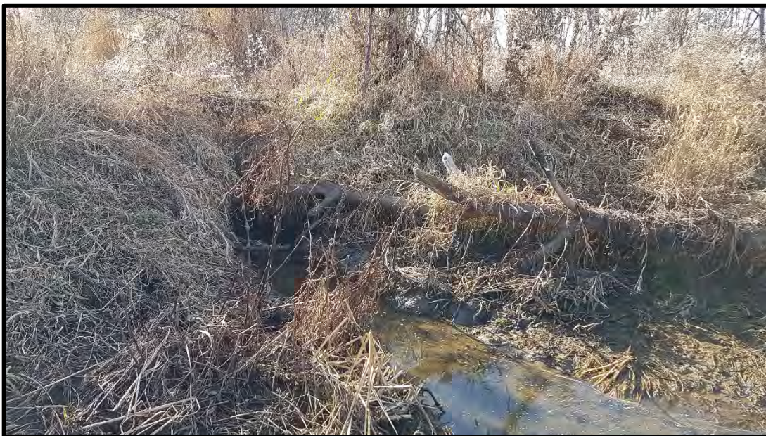
PHOTOGRAPH NO.: 20 FROM: Beaver Dam LOOKING: Downstream
