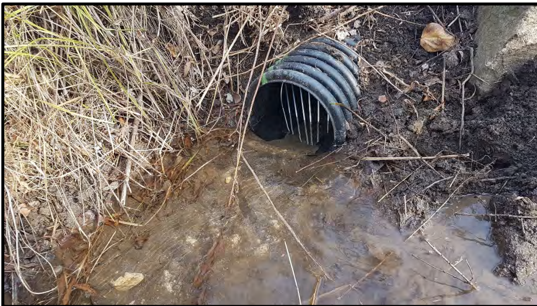
PHOTOGRAPH NO.: 8 FROM: Culvert LOOKING: Upstream at culvert
