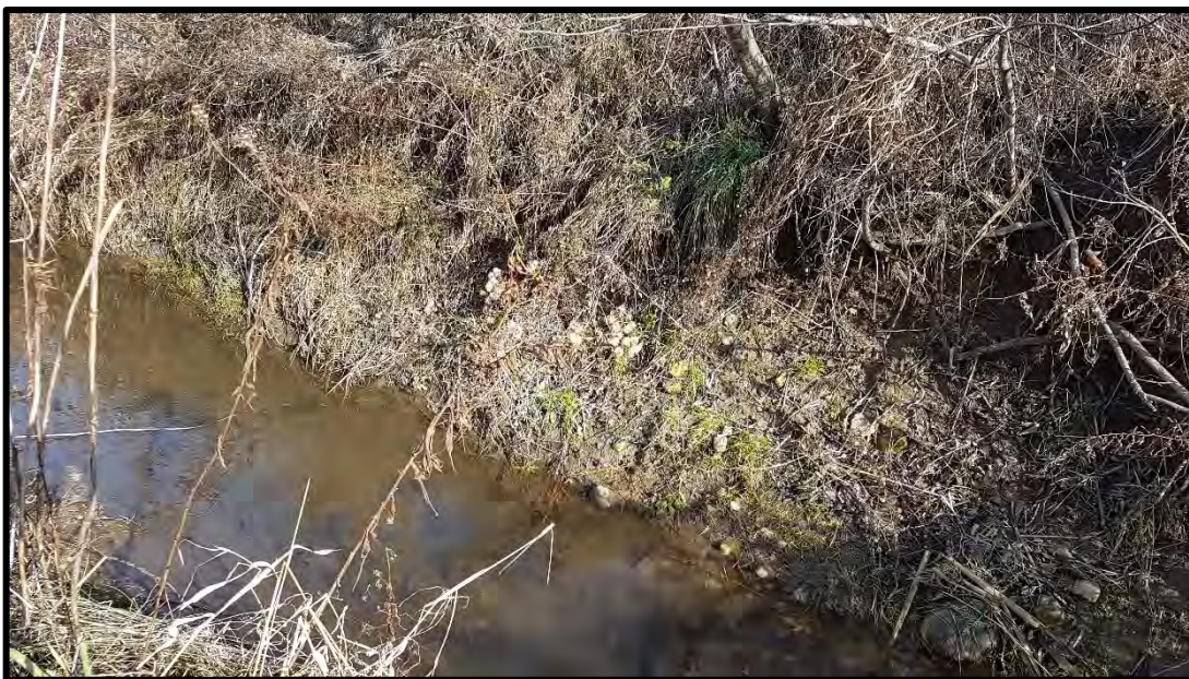
PHOTOGRAPH NO.: 22 FROM: Left bank LOOKING: Onto left bank
