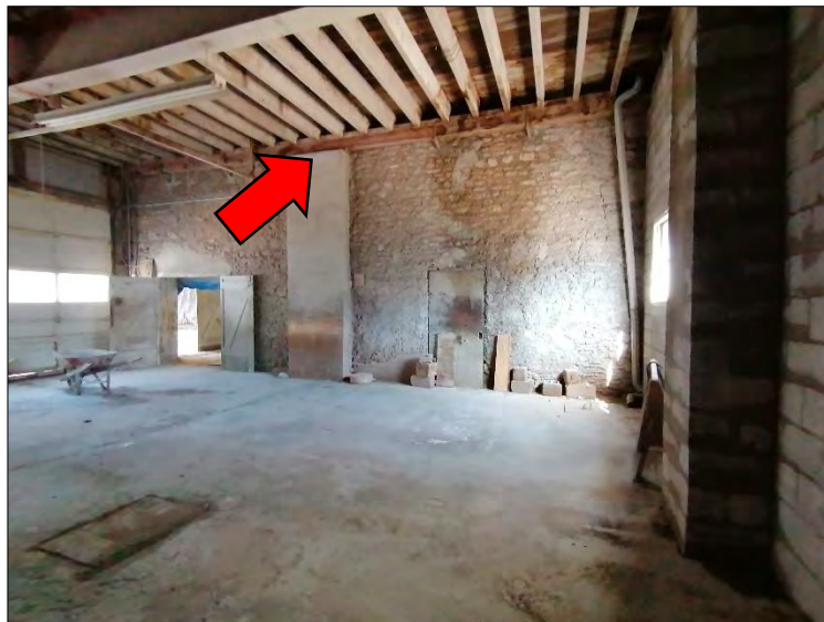
Figures 49 & 50: (above) View of north elevation of historic stone building (Building B) showing concrete carport and location of steel beams on this elevation; (below) View of attachment of western addition to historic stone building (Building B) (Source: MHBC, 2021).
