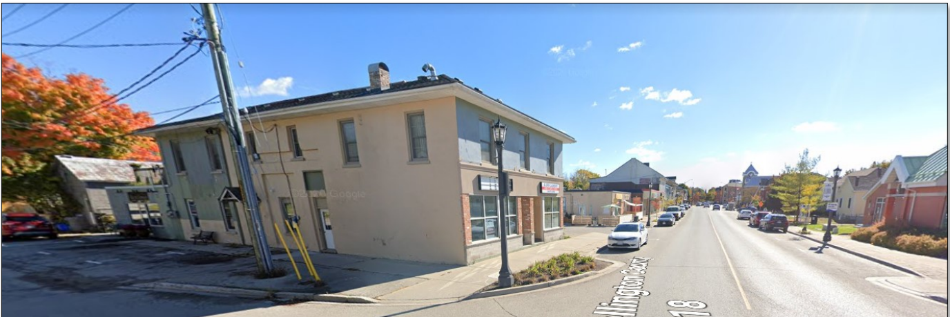
SUBJECT LANDS. LOOKING SOUTH TOWARDS WATER ST (DOWNTOWN ELORA)
