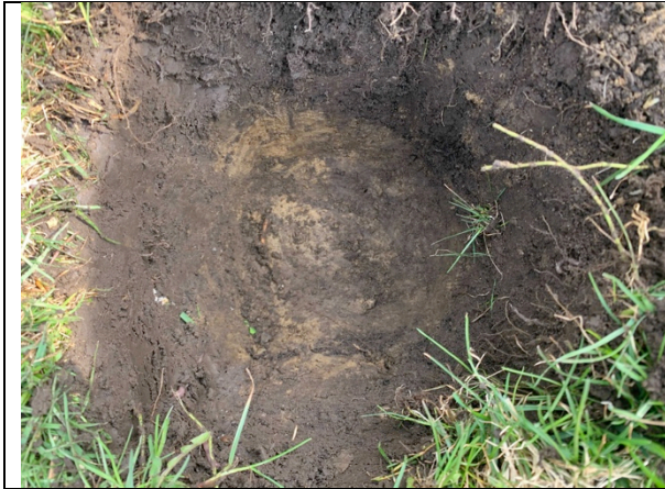
IMAGE 19 TEST PIT IN PROGRESS
