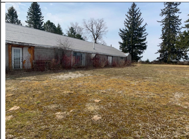
IMAGE 17 SHED AND GRAVEL ON TOPSOIL
